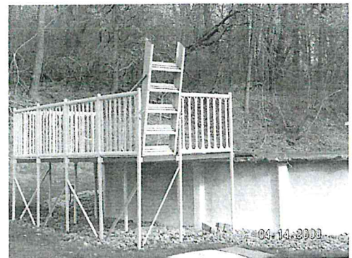
Figure 3. Ladder/stairs that are capable of being swung up and locked into position so that the safety barrier is in place while the pool is not in use. Include label on ladder.
